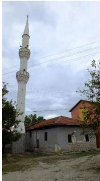
Pic.1. Overall view of Çukur Village Mosque
