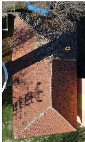
Pic. 3. Roof View
