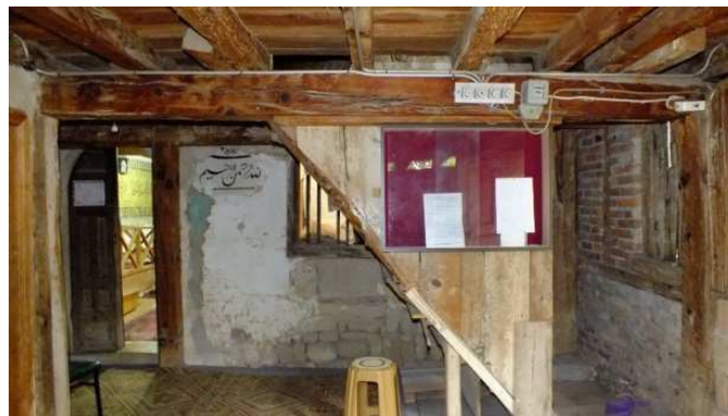
Pic. 6. Additional Section in the North, Ladders to Upstairs
