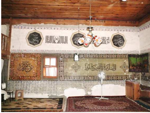
Pic.17. East Wall Second and Third Horizontal Parts
