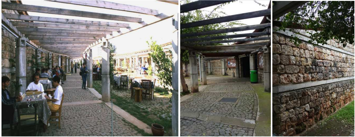
Fig 20: Outdoor stoa and shops in the background (URL 15). Middle: Stoa (Author) Right: Local travertine stone and local wall masonry with precast concrete (Author).
